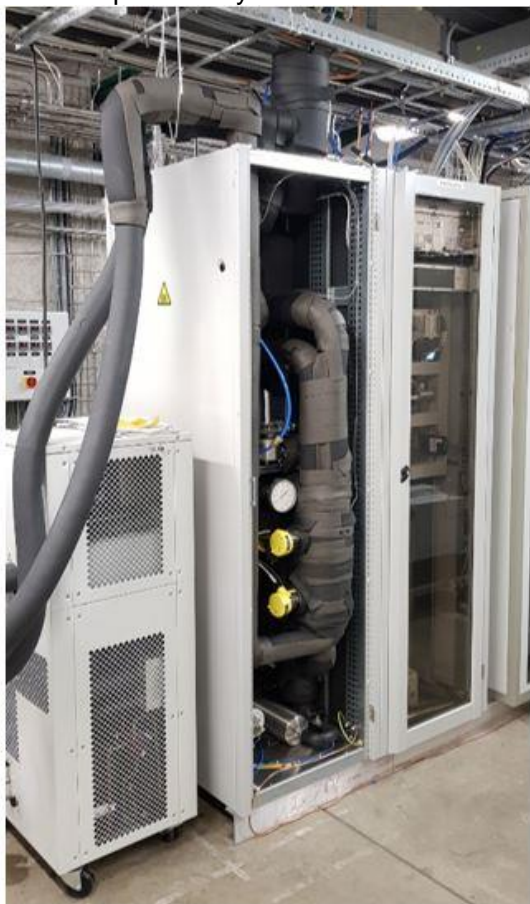
Figure 1: First prototype of the R134a recuperation plant successfully tested recently on the RPC detector system.
