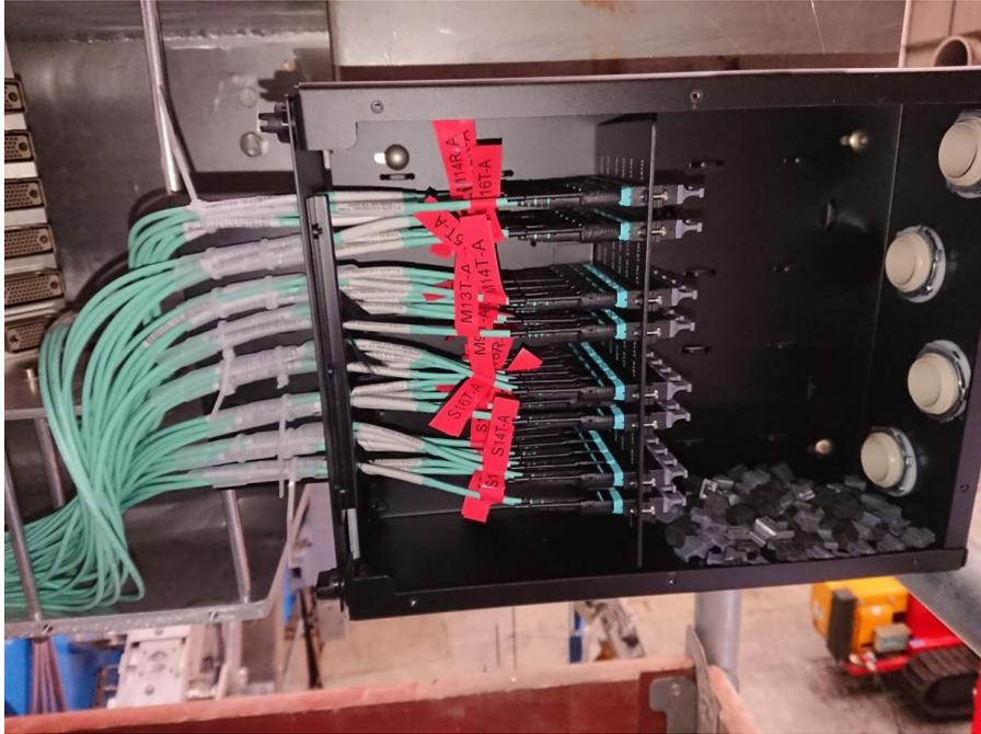
**Figure 3: A fiber connection panel at the edge of the wheels.**
